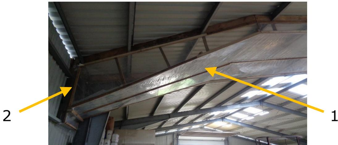
Fig. 2. Air collecting channel covered with polyethylene film: 1 – air collection channel; 2 – connection between the duct and air collection channel
